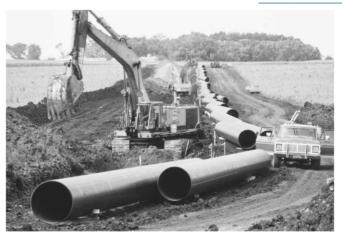
A crane moves soil next to sections of 42-inch pipes to be used for a gas pipeline. (Corbis-Bettmann)
