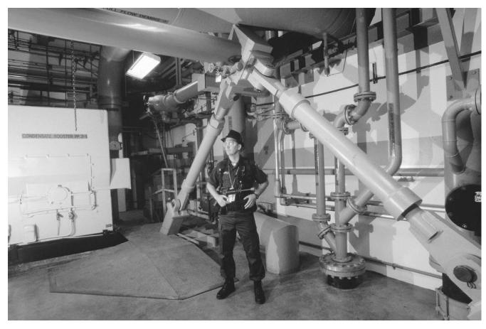
The seismic braces seen here in the Diablo Canyon Nuclear Power Plant reduce the risks associated with an area prone to earthquakes. (Corbis Corporation)
